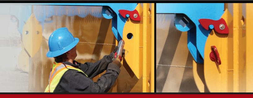
The Gravity Locks engage before the worker enters the area, keeping workers out of danger.
